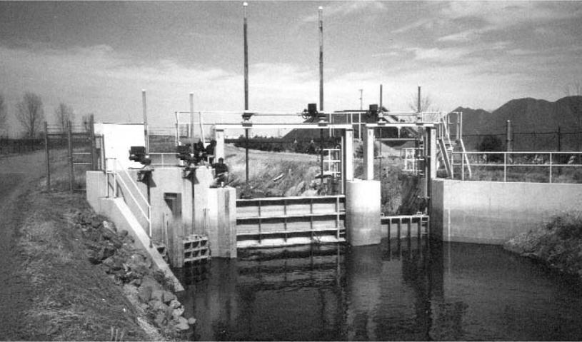
Hydro Gate® roller gates are designed to control flow through large waterway openings where economy and ease of operation are important. They may be designed as either upward or downward (skimmer) opening.
