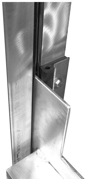
UHMW LINER AND J SEAL ASSEMBLY
