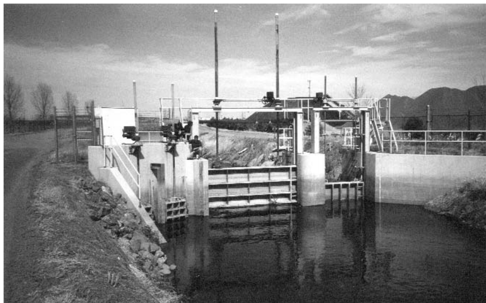
Tandem electrically actuated roller gates.
