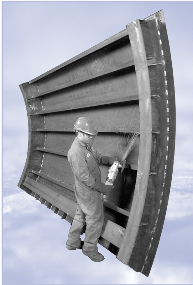
Radial Gate Fabrication
