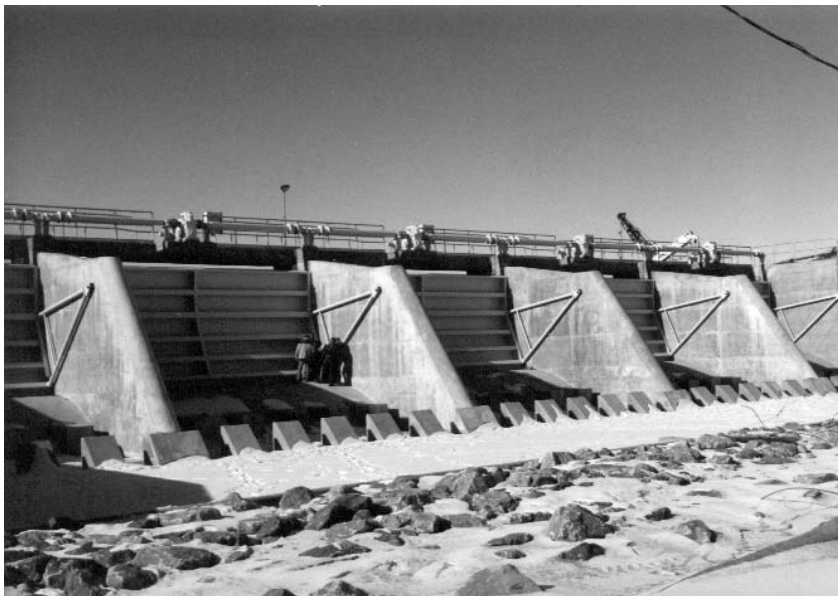
Overflow radial gate installation
